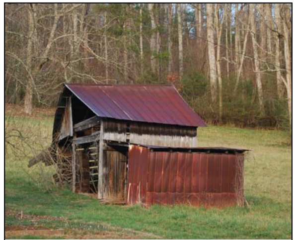
Photograph 13. Frame Equipment Garage
