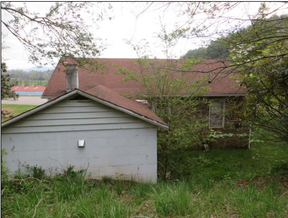
Photograph 9. Rear (West) Elevation
