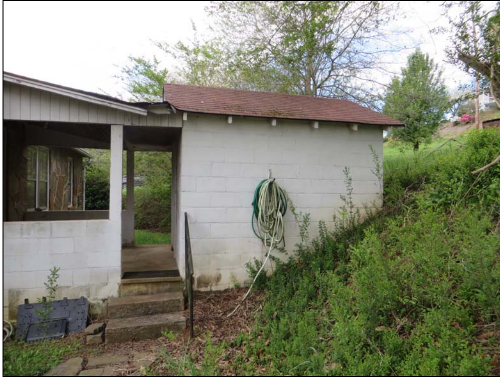
Photograph 10. Concrete Block Utility Room and Breezeway
