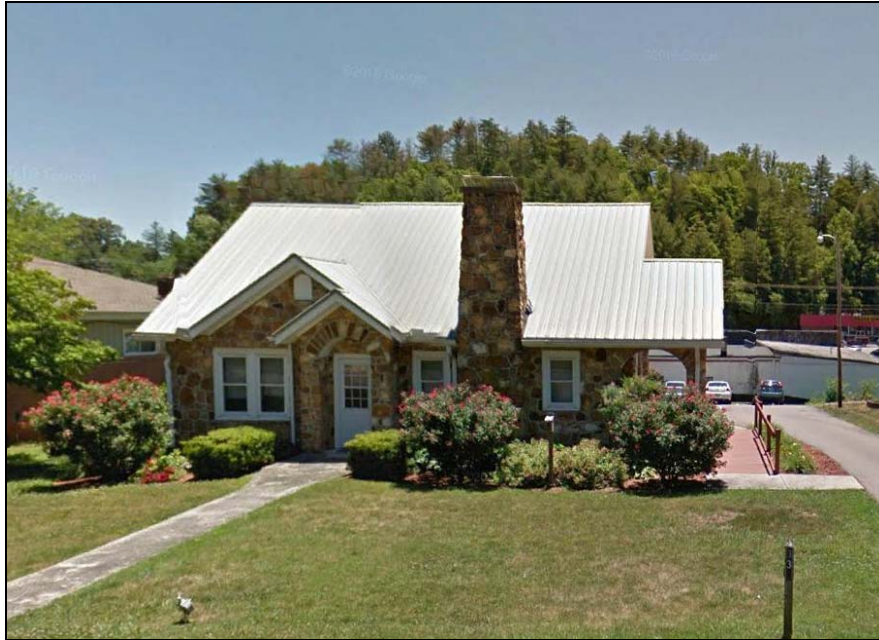
Photograph 16. 330 W. Main Street
